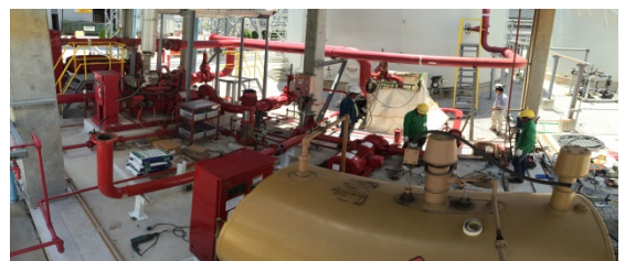
Project Rayong : Fire Pump Installation, Pump Alignment & Commissioning
