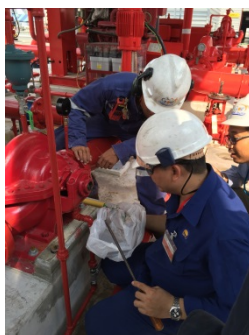
Project Rayong : Fire Pump Installation, Pump Alignment & Commissioning
